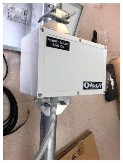
Next mount the Remote Solar Station equipment box to the 60mm Galvanised Pipe using the U-bolts, nuts and washers provided. Locate the box directly below the Solar Panel Mount.
