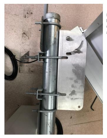
Next mount the solar panel mounting bracket to the 60mm Galvanised Pipe using the supplied U-bolts, washers and screws.
